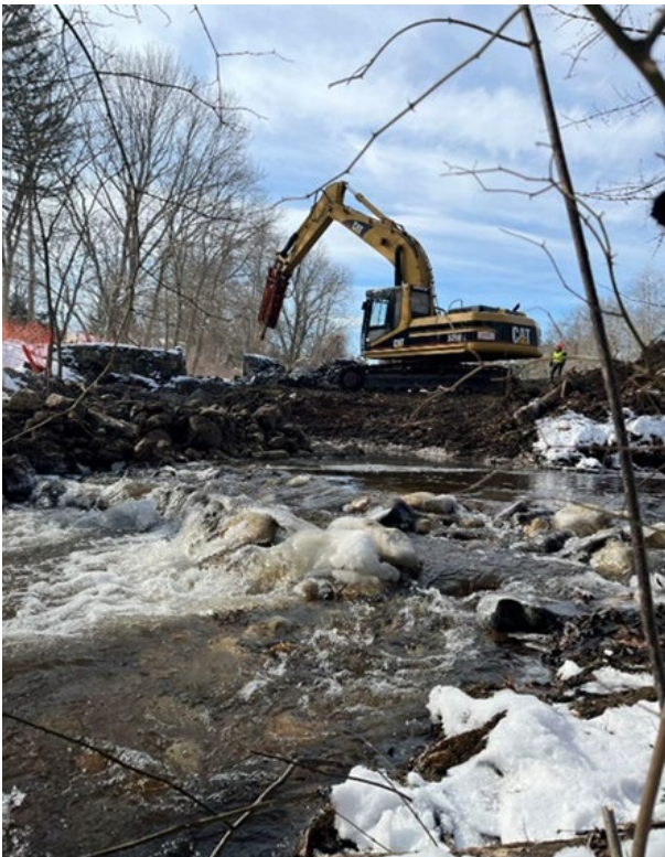
Mill Pond Dam removal. Photo: MADEP.
