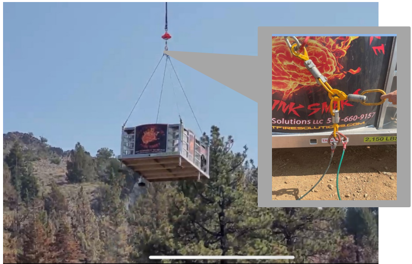
Recommended Rigging for Smart Pumps
